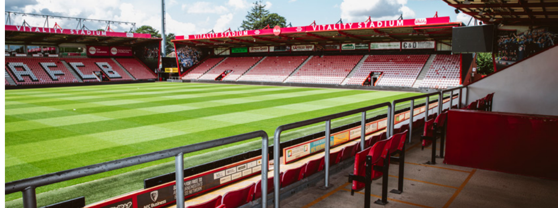
Photo: East Stand Elevated Viewing Platform
