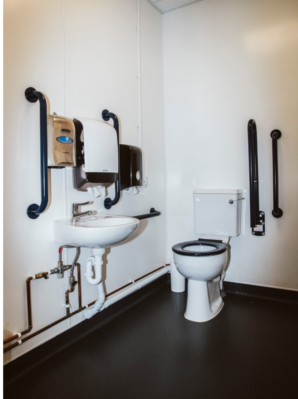
Photo: Accessible Toilet
